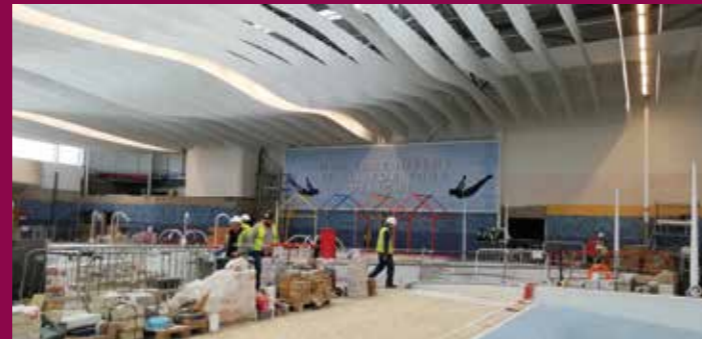
Pool area under construction
