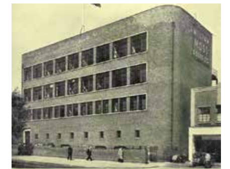
William Moss & Sons Staples Corner office
